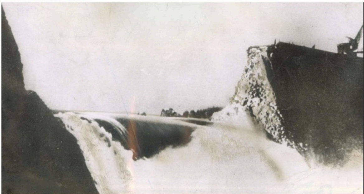
Moehne Dam 5 hours after the attack
